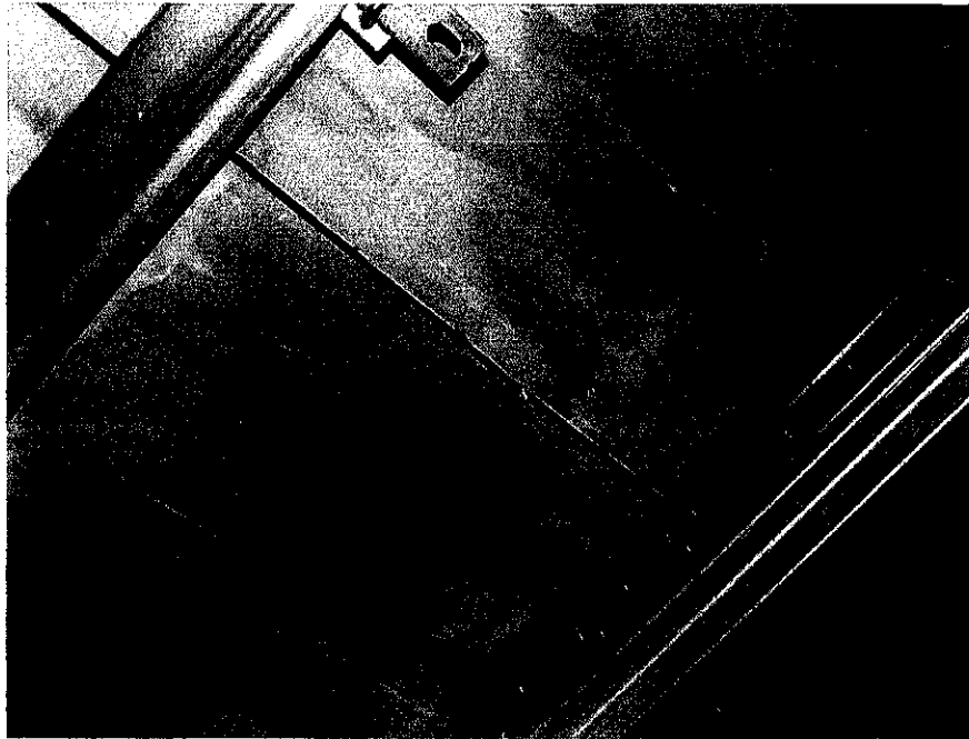
Photograph 7. Missing H-Clip Along Plywood Seam
