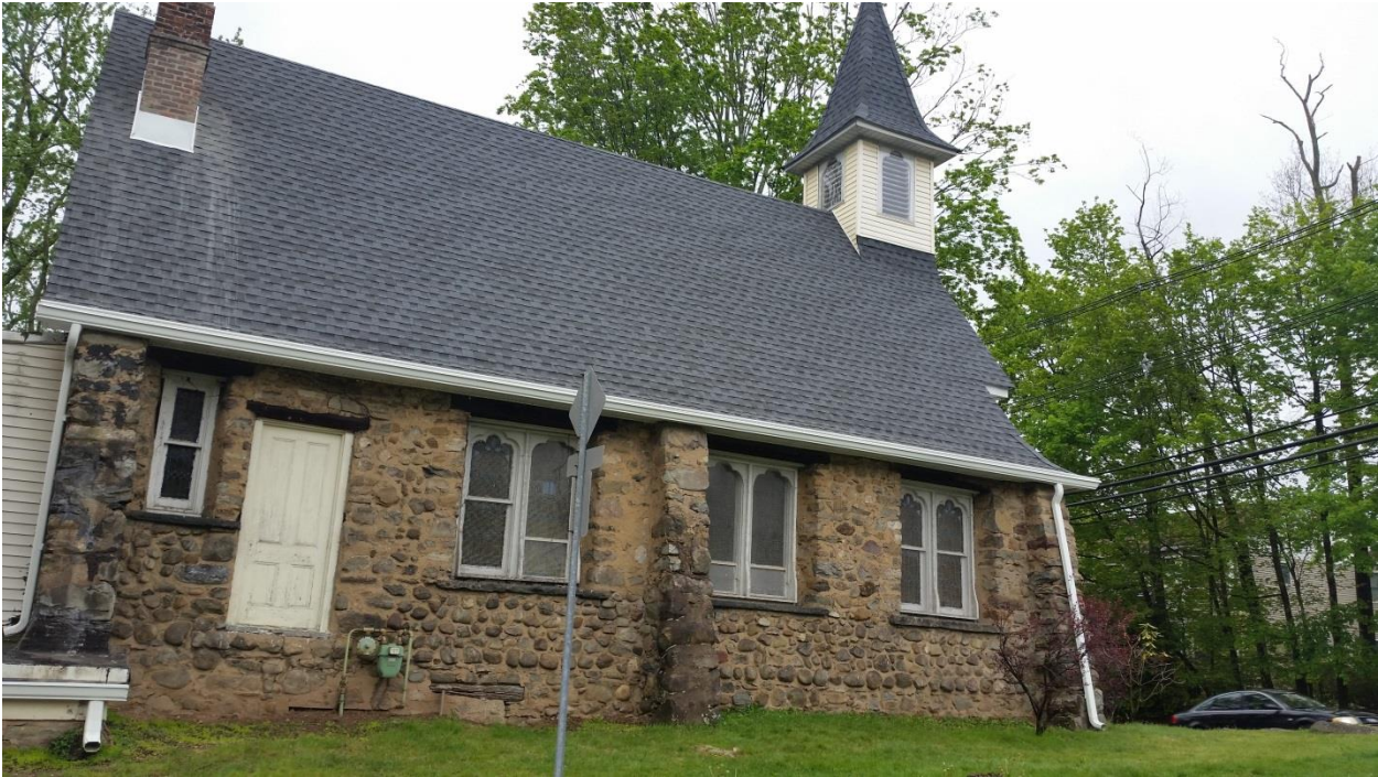
Photo 2: View of historic church from Woodland Road.
